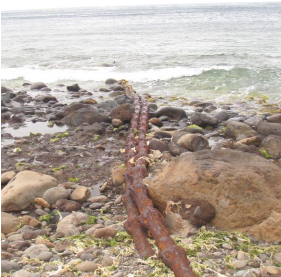
Post-installation remediation work.
