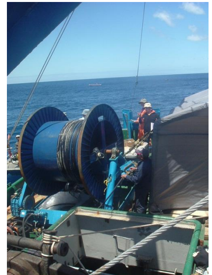
FO cable repair work, Robinson Crusoe Island.
