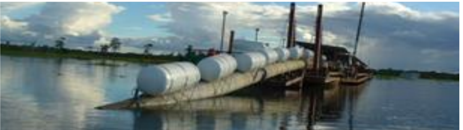
Amazon River gas pipeline.
