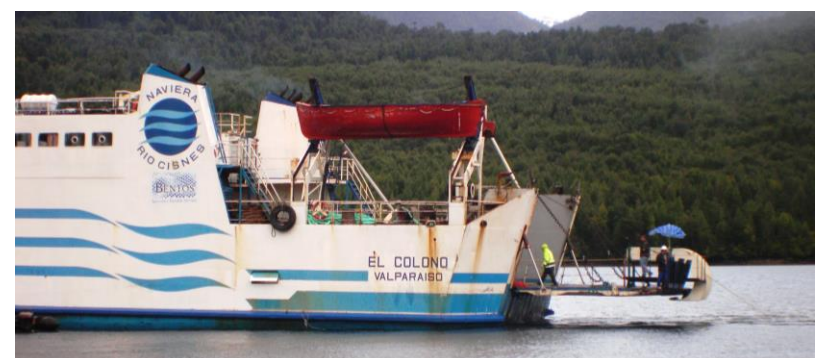
FO cable installation, Patagonia, Chile.
