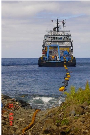
Submarine cable installation, Robinson Crusoe Island.
